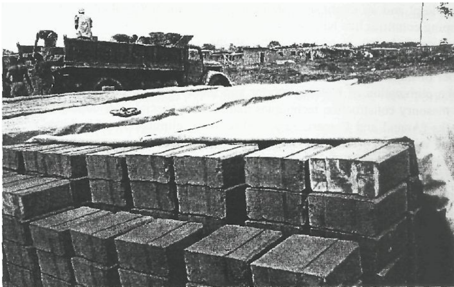
Plate 2: Curing and Stacking of Interlocking Blocks
